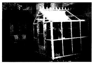
Jan wanted a greenhouse after she retired and had time to propagate indoor plants. Aluminum contractors wanted \$5000 for a 10' by 12' dirt floor unit. I built a wood and plexiglass unit with brick floor, heater and powervent for just over \$1000.00.
